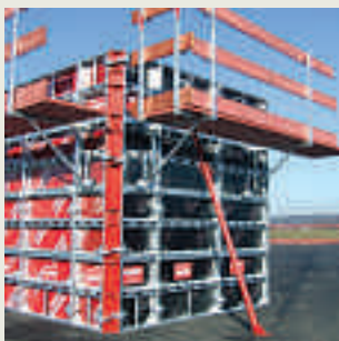
Concreting brackets with guardrails
